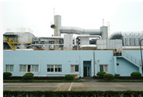
Combustion-type VOC treatment equipment, TRJ (China)
