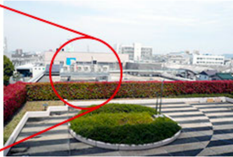
Moved outdoor units on the roof of old R&D headquarters
