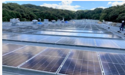
Newly installed solar panels Tokai Chemical Industries, Ltd.
