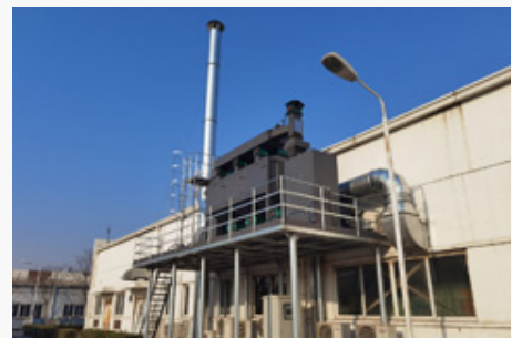
Combustion-type treatment equipment for gas generated by vulcanization Tokai Rubber Moldings (Tianjin) Co., Ltd. (China)
